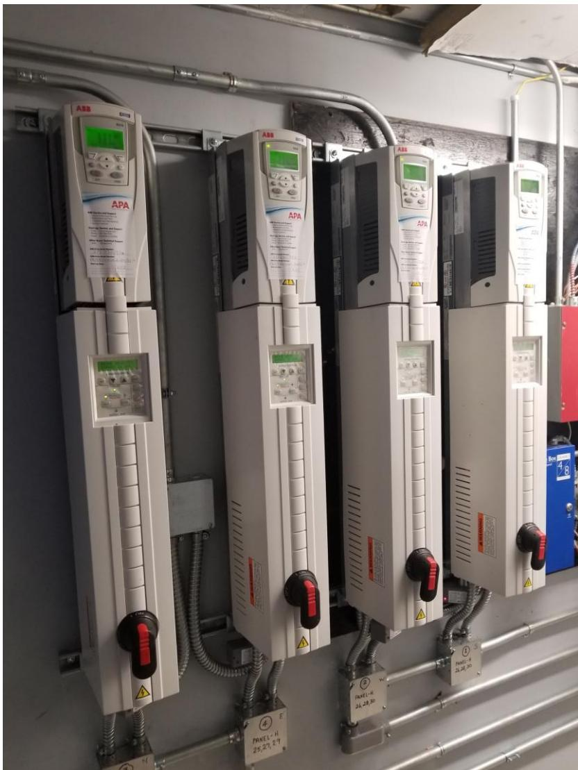
VFDs are a type of motor controller that can cut down energy costs by controlling the speed of electric motors.
