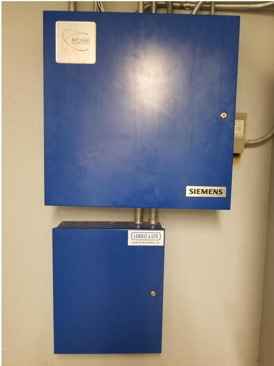
*Siemens control panels are being installed along with Variable Frequency Drives throughout campus. These systems allow for better energy management of the HVAC systems of campus buildings.*
