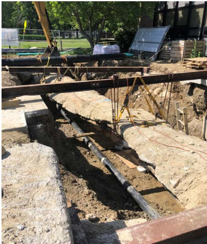
***Steam Distribution replacement – More piping being installed under existing piping and concrete encased conduit (Alger).***
